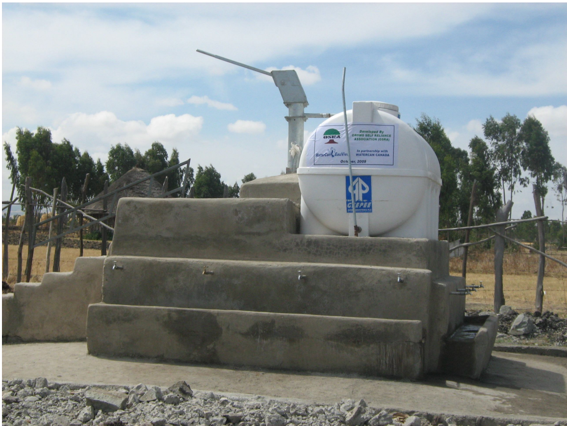
Photo: wellhead and distribution point with 11 facets at Keta Insilale
